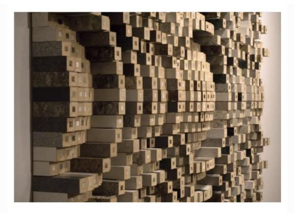
This is a close up of a <u>2 dimensional QRD panel</u>. While the panel was constructed using reclaimed wood scraps, the mathematical pattern behind the design of the panel also reduces <u>slap</u> or flutter echo. The goal is to reduce the room coloration to the sound quality without making the listening room an <u>anechoic chamber</u>.
