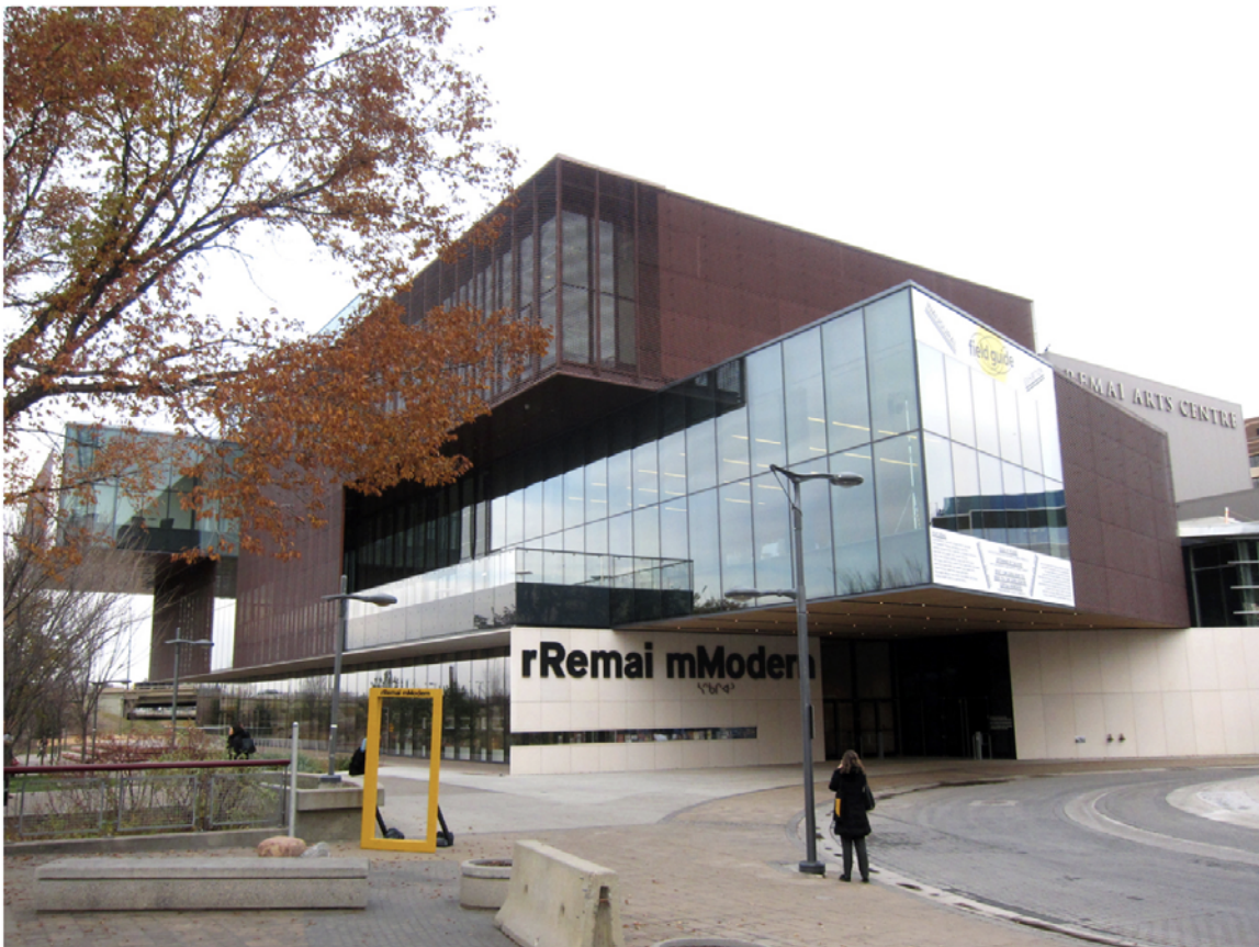
Exterior of the Remai Modern in Saskatoon, designed by architect Bruce Kuwabara (all photos by the author for Hyperallergic)
